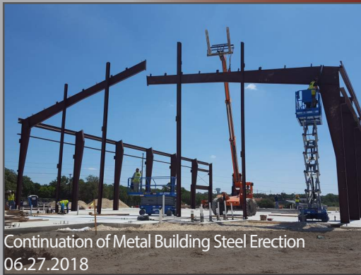
Continuation of Metal Building Steel Erection 06.28.2018
