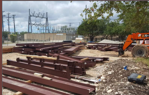
Pre-engineered Metal Building Materials Delivered & Stockpiled _ 06.20.2018
