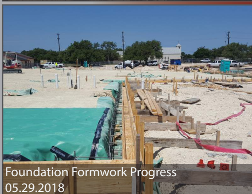
Foundation Formwork Progress 05.29.2018
