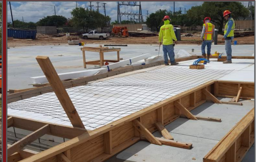
Worship Hall Stage/Altar formwork 06.20.2018
