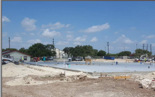
Building Foundation & Floor Slab 06.11.2018
