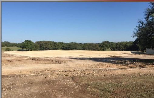
Building Pad Finalized 04.15.2018
