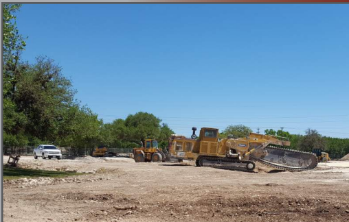
Trenching Equipment Delivered to Site 04.21.2018
