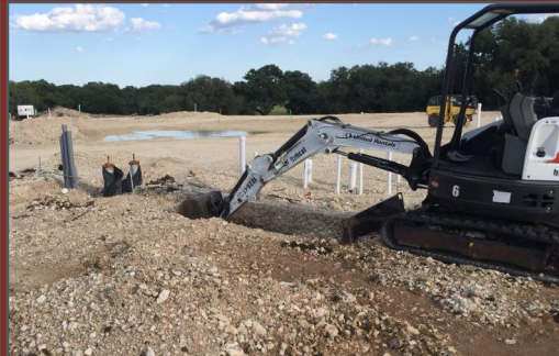
Trench for Building Utilities 05.05.2018
