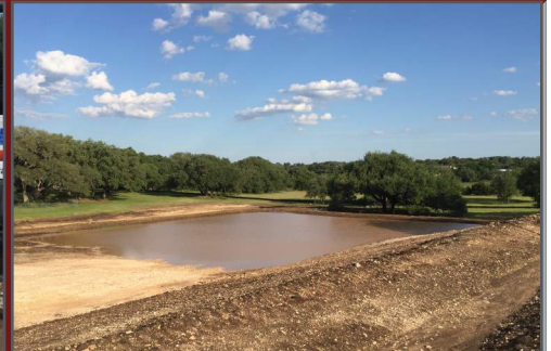
Removal & Stockpiling of Topsoil at Future Detention Pond _ 05.05.2018
