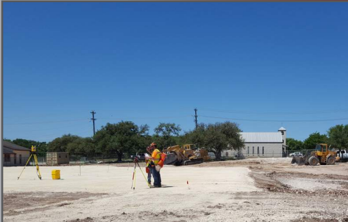
Establishing building corners 04.24.2018
