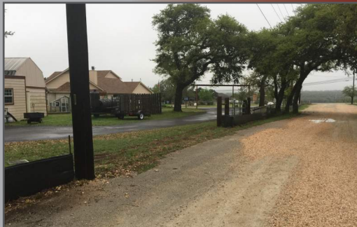
Silt Fence Installation 03.28.2018
