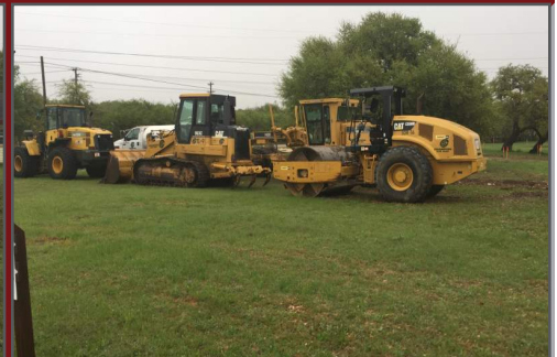
Sitework equipment Delivered 03.28.2018
