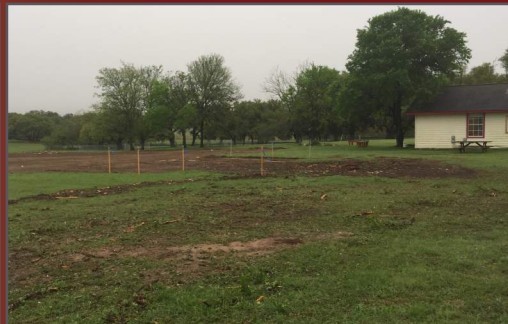
Removal & Stockpiling of Topsoil 03.28.2018
