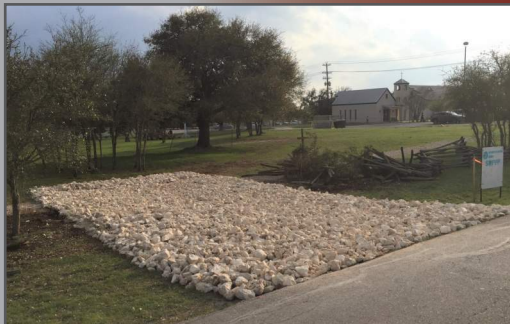
Construction Entrance Installed 03.17.2018
